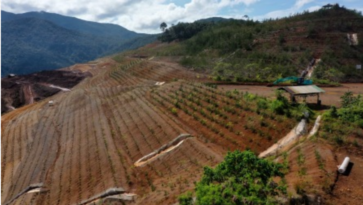
PHOTO: BNC installs 1,506 coco-coir nets at the Berong mine site as of March 2024, 29% higher than its two-year target of 1,166
