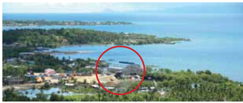
13MW Diesel Power Plant in Mobo, Masbate
