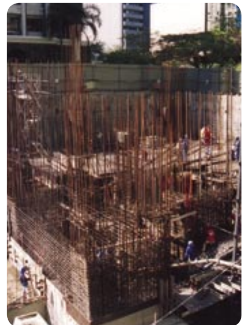
Construction at the Four Seasons in Salcedo, Makati City
